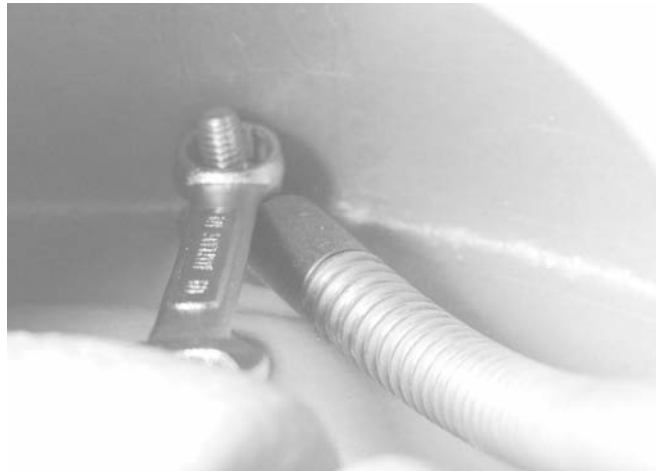
Figure 14 – Removing Pigtail Anchoring Bolt
