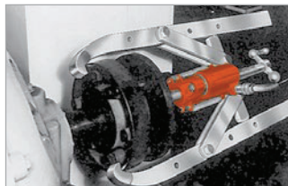
Flexible coupler is removed from electric motor shaft with 2-jaw puller.
